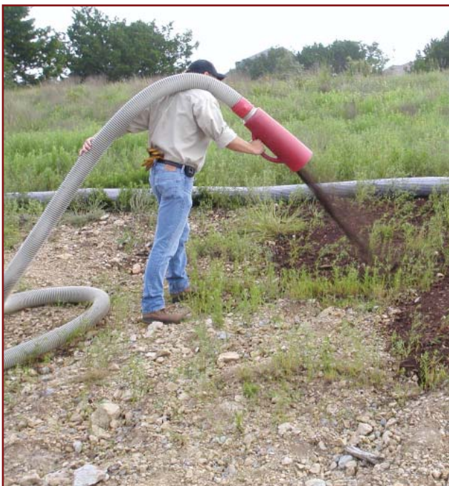
Smaller units like this pneumatic/blower, propel compost through a wide hose which can be directed around plants and other objects. It also works well when applying compost to slopes and roadsides.
