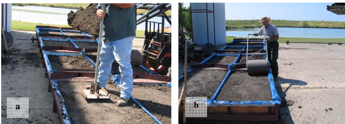
Figure 2. Soil compaction with hand tamping (a) and soil leveling with a drum roller (b).
